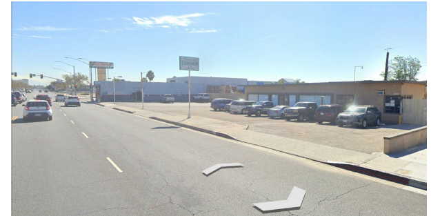
Figure 5.3 Conditions on Holt Avenue. excess vehicle entrances, and wide street widths Photo Source: Google
